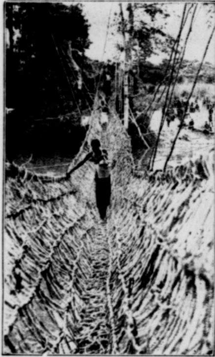
Suspension bridge of vines built by natives across the Luletu River, over which Bishop Lambuth and his caravan passed. Central Africa.
