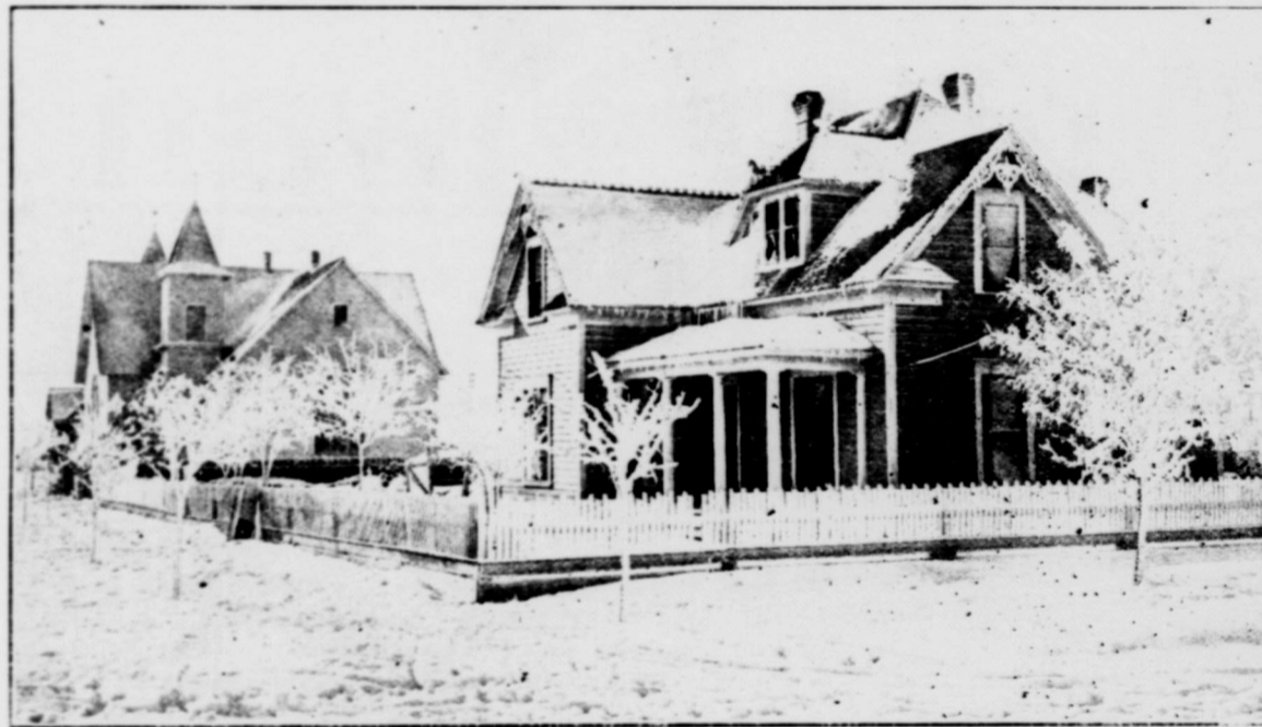
METHODIST EPISCOPAL CHURCH, SOUTH, AND PARSONAGE
