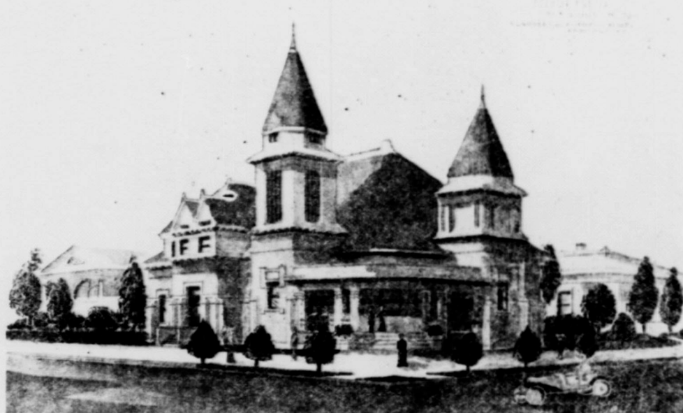
The above is our new Methodist Church at Rosebud, Texas, modern in all its arrangements and just completed by Rev. James F. Carter, the pastor of the Church, and his loyal Building Committee. It is no longer on paper, but is a reality. It is a two-story veneer building, built of buff brick, with memorial windows. The main auditorium seats 400, the Sunday-school room 300. The main auditorium and the Sunday-school room can be separated by a hoisting partition, lowered and raised by an iron crank. It has six modern Sunday-school classrooms and a Primary room which can be closed to the main Sunday-school by accordion doors. It has a Trustees', Board of Stewards' and a choir room in the rear of pulpit rostrum. There are two south vestibule entrances, porch, with concrete floor and steps; a west vestibule entrance, hooded, and concrete steps. In the vestibule this entrance is a closet. An east entrance from the ground, concrete floor and elevated wooden steps to the main auditorium and Sunday-school. A basement for the heating furnace. Upstairs: A pastor's study, large and commodious Philathea and Baraca rooms, an assembly hall, a home mission room, with a cloakroom. Its electric lights and equipments are the best and most modern.
