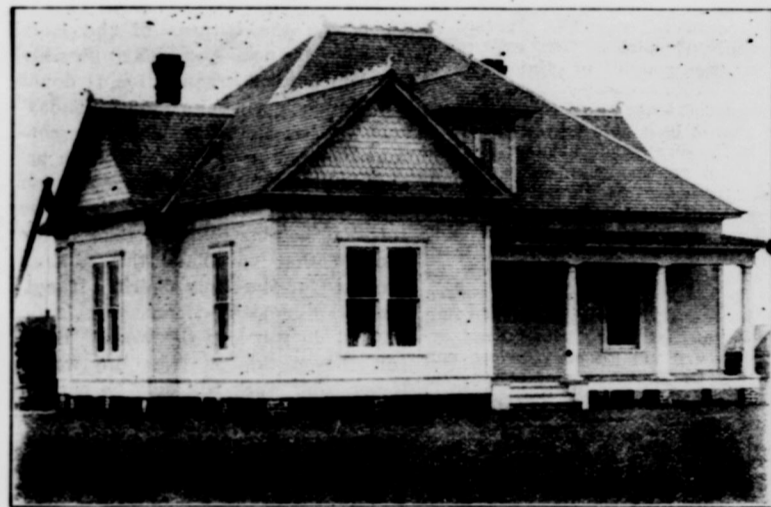
Parsonage at Knox City, Texas. Rev. Zoro B. Pirtle, P. C. This new parsonage has been projected and completed since conference at Brownwood, Texas. The contract price was $1200 cash. It is a beauty, built upon an elevation from which the water runs in every direction.
