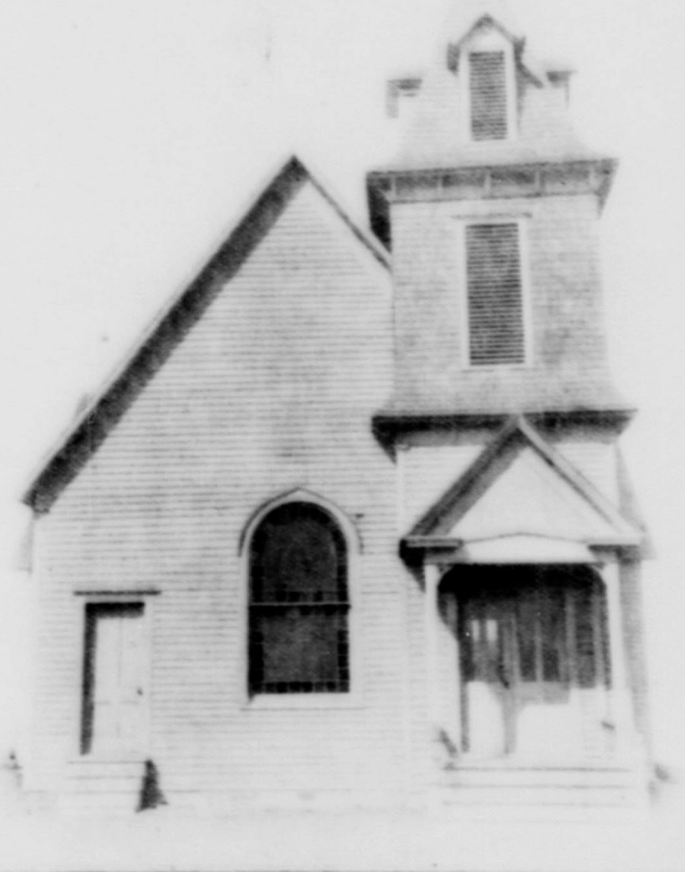
OUR CHURCH AT MANGUM. The above is a picture of the Methodist Episcopal Church, South, at Mangum, Oklahoma, which was dedicated October 15, 1899. The main body is 30x40 feet, with a T 30x40 feet, built and modeled after the very latest of church architecture, has stained glass windows, and is neatly finished and furnished throughout.
