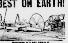
PONY SAW MILL. Can be run with a 10 or 12 Horse Threshing Engine, will saw 4,500 feet in day. BAGLE MACHINE WORKS,
