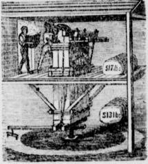
PRICE COMPLETE. Screw or pin. 4 inches, solid wrought iron acking box, 9 feet deep. Simple, strong, durate and guaranteed to pack a 500 fbs, bale. Send or circular. Manufactured by H. DUDLEY COLEMAN & BRO., New Orleans, La
