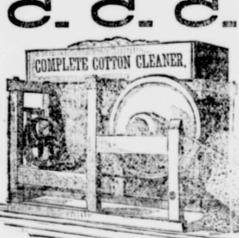
The Complete Cotton Cleaner, a New, Valuable and Moneymaking Machine to every Cotton producer or ginner,-thoroughly removes all DUST, DIRT, SAND and light Trash from cotton before ginning, and improves the quality of the lint from one to our grades.
