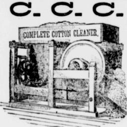
The Complete Cotton Cleaner, a New, Valuable and Moneymaking Machine to every Cotton producer or ginner,-thoroughly removes all Dust, Digt, Sand and light TRASH from cotton before ginning, and improves the quality of the lint from one t
