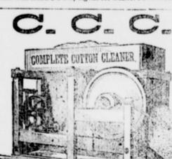
The Complete Cotton Cleaner. a New, Valuable and Moneymaking Machine to every Cotton producer or ginner,-thoroughly removes all Dust, Dirt, Sand and light TRASH from cotton before ginning, and improves the quality of the lint from one to four grades.
