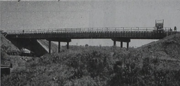
Construction on overpass viaduct over E-W railroad tracks in Baird.
