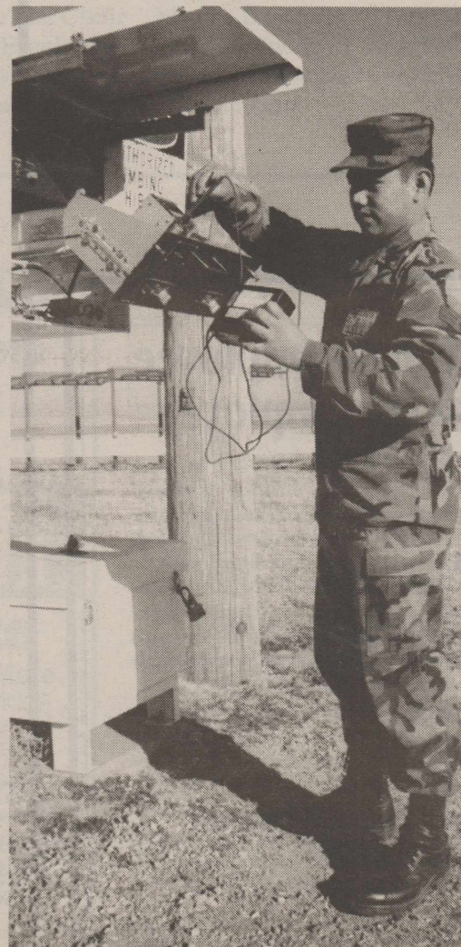
Airman 1st Class Joseph Dungo performs routine maintenance on the far field monitor south of the runways.
