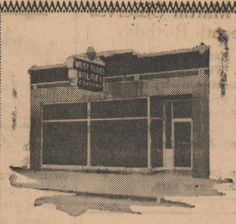
Recently remodeled WTU office at Haskell
