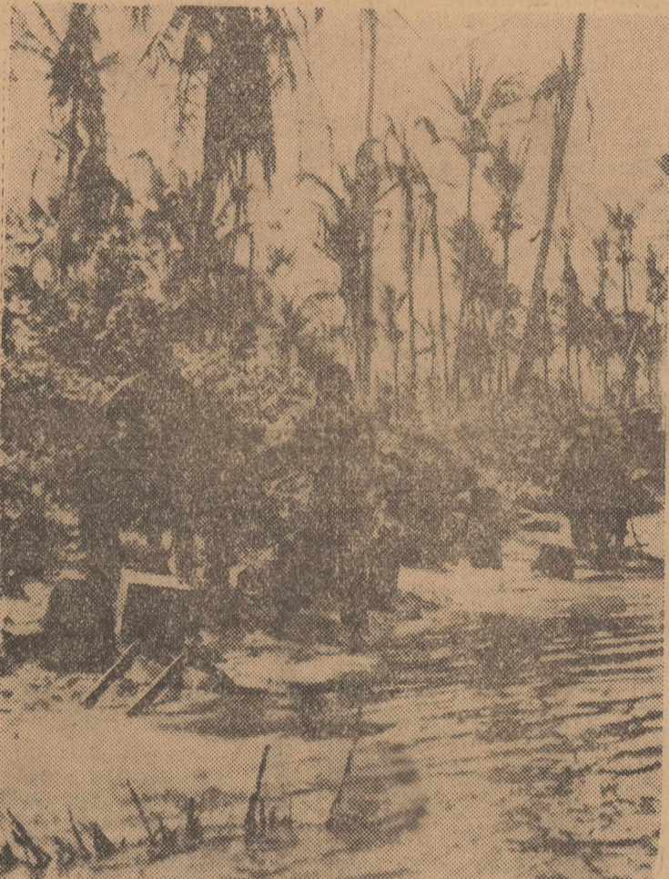
Fifty caliber machine guns are installed on the beach at Arawe in New Britain. (Passed censors)
