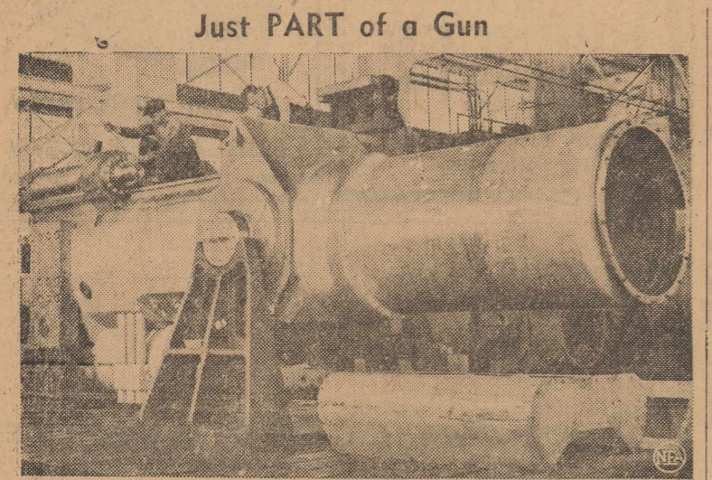
Just PART of a Gun Looking like a giant cannon, but actually only a part of one, the 25-ton mass of steel above is the stationary housing for the recoil mechanism of a 16-inch Naval gun. Destined soon to blast the foe from one of our new battlewagons, it is getting a final check at the Westinghouse Naval Ordnance plant at Louisville, Ky.
