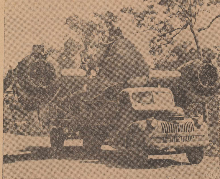
This strange manner of vehicle is just a big truck ferrying a disabled Australian Beaufighter to the repair shop after it came in on one motor and made a belly landing. The Aussie fighter squadron in northwest Australia has downed 60 Jap planes.
