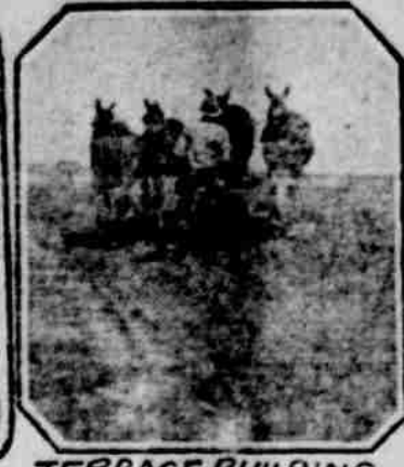
TERRACE BUILDING SPUR STATION
