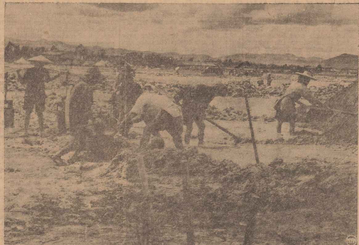
(U. S. Army Air Force Photo From NEA) Fashioned by the hands of determined Chinese workers in a sheltered valley, the airfield you see here under construction is now being used as a base to bomb the Japs. Mud was used to bind the rocks together and form a level surface as the Chinese youths and women toiled with crude tools of bygone centuries to build a base for modern bombers.
