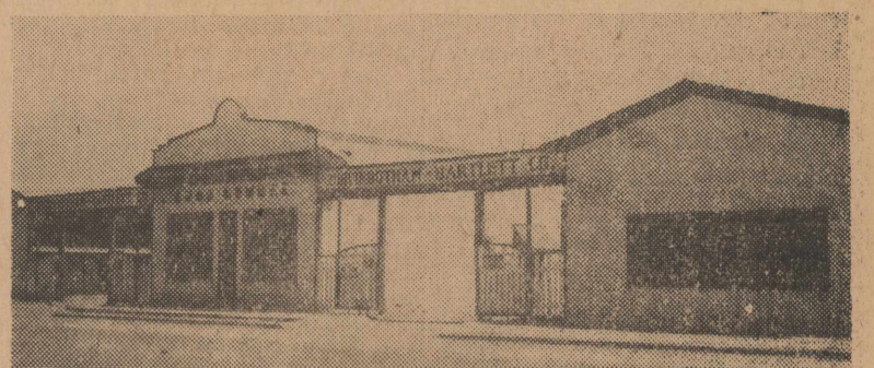
Despite wartime shortages, the Higginbotham-Bartlett Company, 217 West Missouri Avenue, still is able to offer good lines of hardware and building supplies. A complete glass department is operated by the company.
