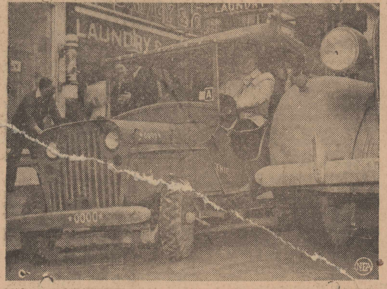
Midget model jeep "Squeekie," which Oakland iron works superintendent William Mason built for his son's Christmas present last year, has been reclaimed by the family to combat rationing troubles. Two-cylinder motor gets 35 miles to the gallon; small size "implementation tires" are unrated.
