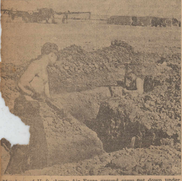
Members of U. S. Army Air Force ground crew get down under the ground with pick and shovel as they dig slit trenches at an airfield in Tunisia. Ditches are used to digge bombs and to drain the field when it rains. Note big warbird in background.
