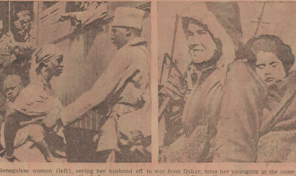
Senegalese woman (left), seeing her husband off to war from Dakar, totes her youngster in the same manner as the Indian woman shipyard worker at Pictou, Nova Scotia.
