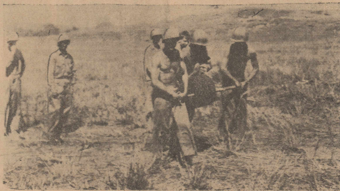
Getting set for the Jap attempt to retake Guadalcanal which they knew was sure to come, these Marines string barbed wire around gun emplacements which guard the sea approaches. (U.S. Navy Photo from NEA Telephoto).
