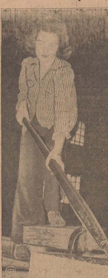
One of more than four thousand women now lumbering in the Northwest, Mildred Mathers, 19, handles big timbers with a peavey.
