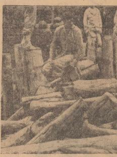
Building an anti-tank "crib." Upright logs are packed with dirt and chunks seen in foreground.
