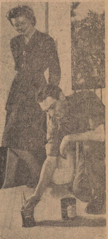
Painting is a good investment, it prevents the deterioration of wood and reduces upkeep costs. It is especially important for surfaces that get hard wear, such as a porch floor.
