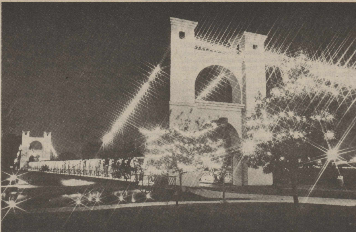
The Waco Suspension Bridge was the longest of its kind in the nation when it was built back in 1870. Thousands of cattle and numerous wagon trains passed over the structure in its heyday, and the famous Brooklyn Bridge in New York was patterned after it. The 475 ft. bridge is still used today, but only as a pedestrian crossing. Tourism Division, Texas Dept of Commerce photo.
