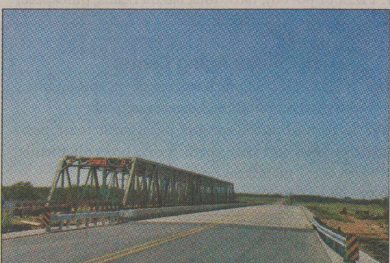
A north to south view of the newly completed SH-6 Bridge in Knox County. The old bridge is also visible and will remain intact for historical purposes. The WPA constructed the Original bridge in the 1930's.
