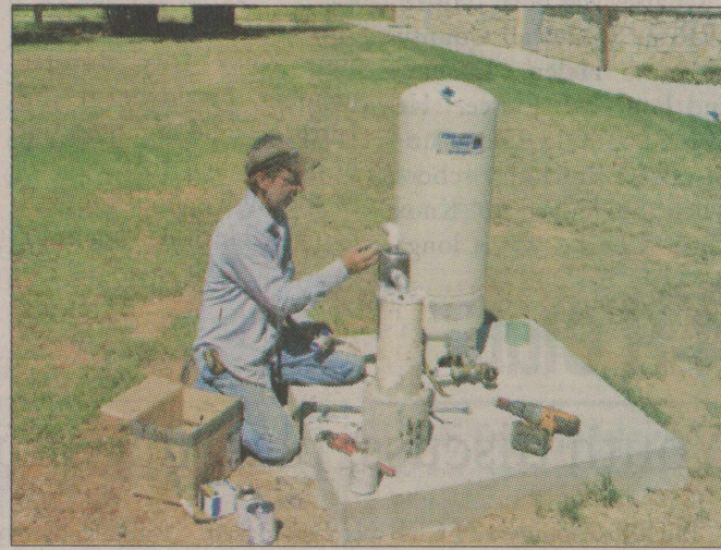
Charlie Fetsch of Decker Electric Co. installs the equipment.
