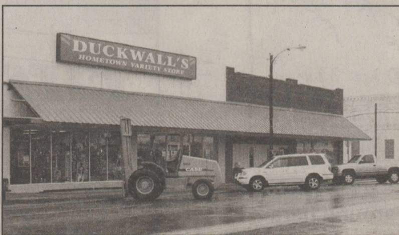
New, vibrant red awnings stretch from the Fitness For Life Gym, Duckwalls and the Art Stall and Frame Shop
