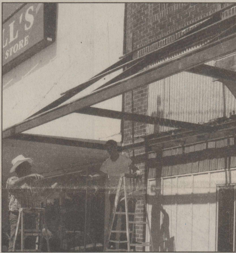
In the beginning stages — Tearing down the old awnings
