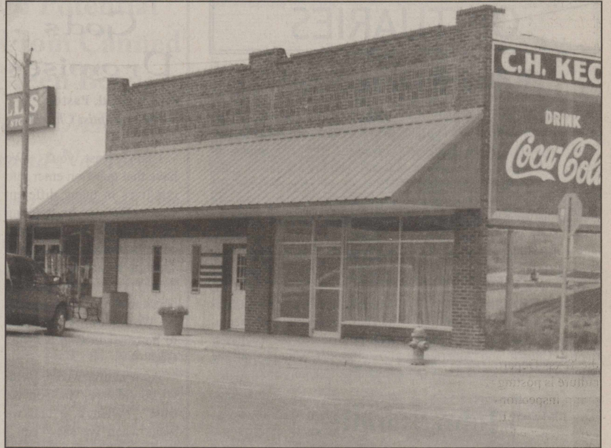
The first of the new awnings was completed before the watermelon festival as planned. The red corrugated tin awning with white underlay was erected above the doorway of the Fitness for Life Gym.
