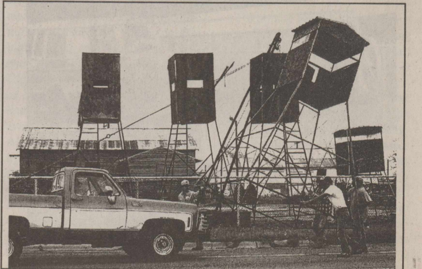
Local crew's clean up after storm.
