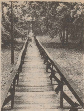
The Rusk footbridge at 546 feet long is thought to be the longest of its kind in the nation. Built in 1861 for crossing a wash during the rainy season, the bridge is located two blocks east of the Rusk town square in northeast Texas. Texas Tourist Agency photo.
