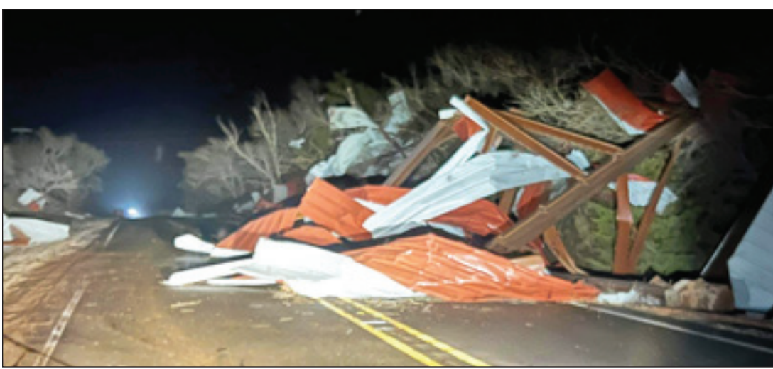
STORM DAMAGE: This is the hay barn belonging to Billy Buckingham after a storm passed through about midnight Sunday. The barn is located one mile east of Kelton. Reported to have been an EF1 tornado. More pictures on page 6.
