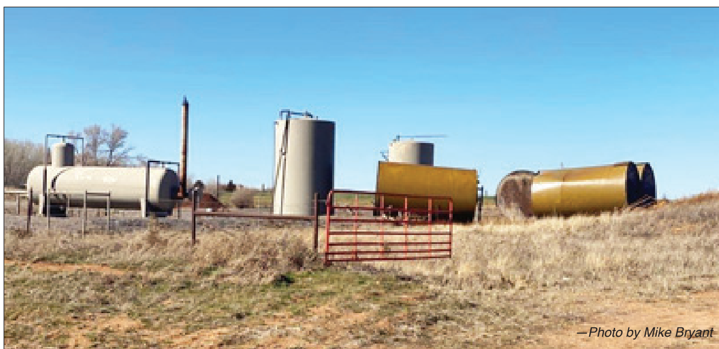
Tanks overturned east of Kelton by storm east of Kelton
