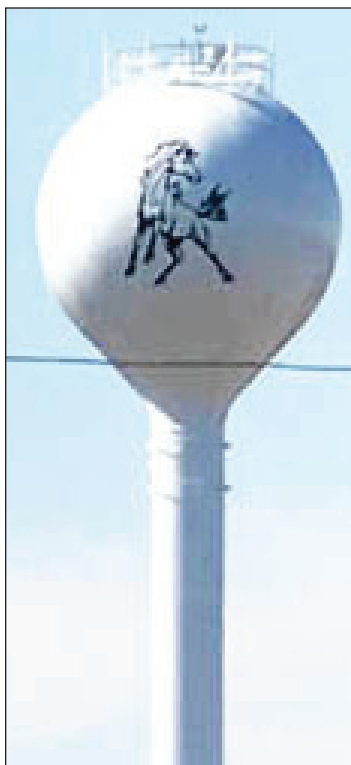
The Wheeler Mustang decorates the new Water Tower. The pumps have not been turned on.
