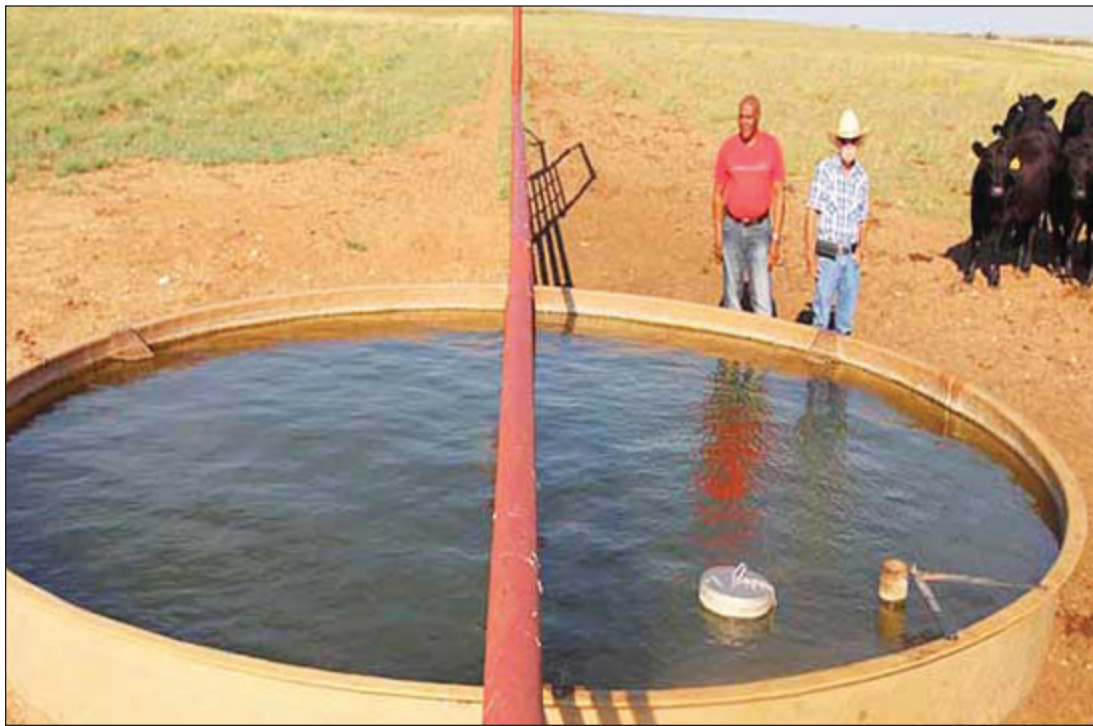
Fred Allison, earth team volunteer (right) and Calvin Devereaux, district conservationist (left) of Wheeler work together on watershed dam rehabilitation in their county
