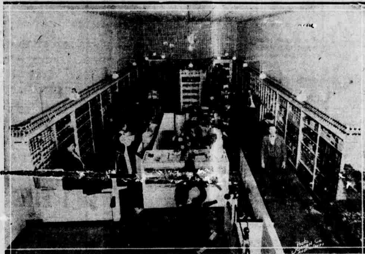
Interior of the New "M" System Store
