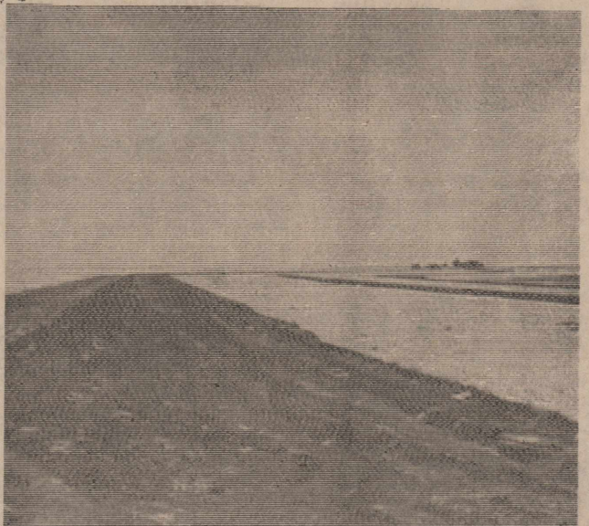
A total of 49,831 feet of terraces were installed in 1982.
