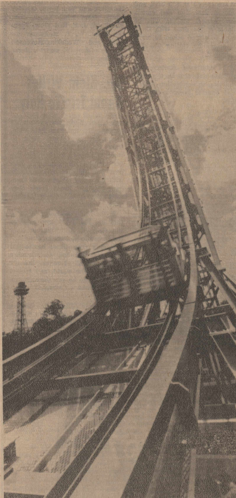
A REAL CLIFFHANGER —The world's first total freefall ride, the Texas Cliffhanger, is in operation at Six Flags Over Texas. The 2.1 million dollar ride carries park guests 128 feet into the sky and then drops them ten stories at freefall speed. Riders then glide to a stop through a computerized braking system at the base of the L-shaped structure.
