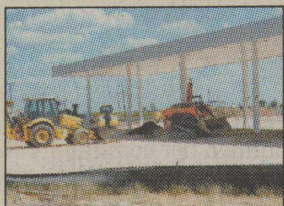
WORK CONTINUES AT THE CROSSING
