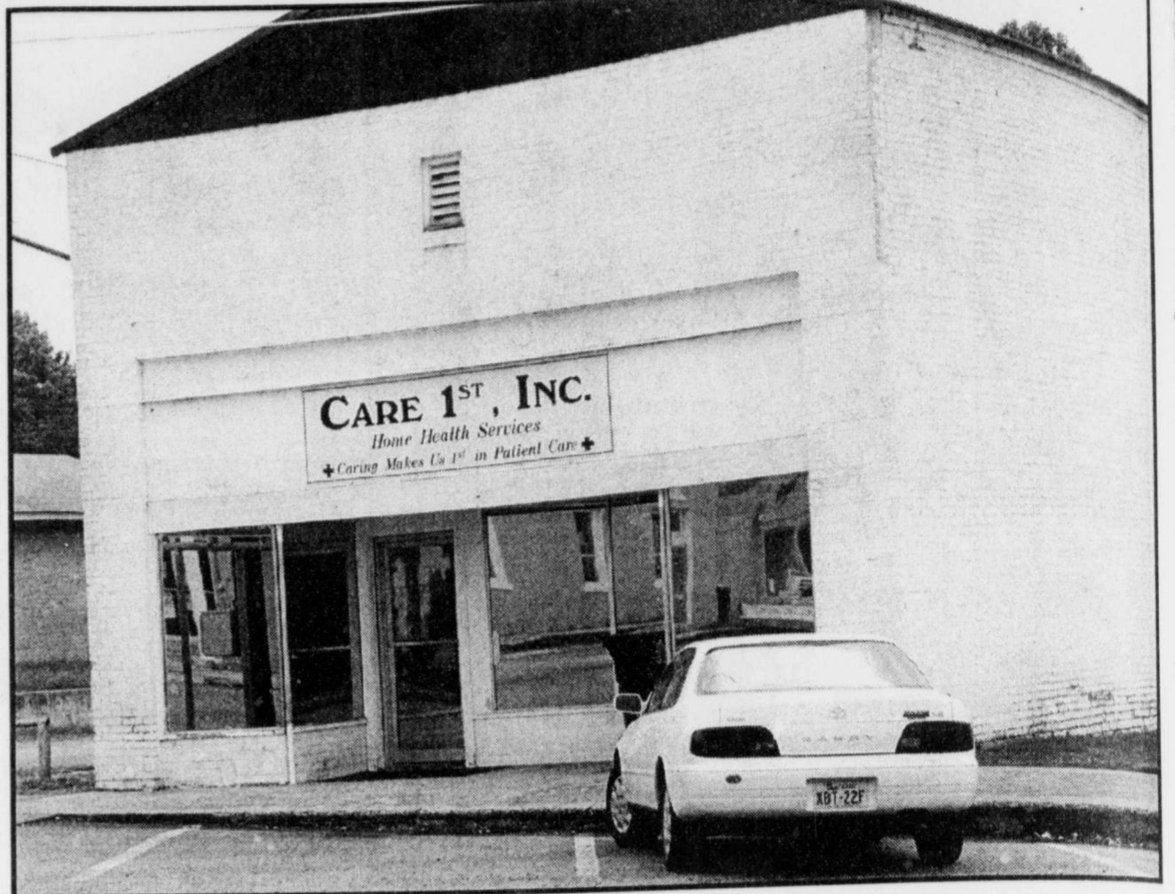
REPAIRS MADE- The Care 1st sign in Bogata fell from the building this past week which led residents to question if the business was still in operation. The sign has been repaired and the business hopes everyone is aware they are still in operation. (Staff Photo Nancy Brown)
