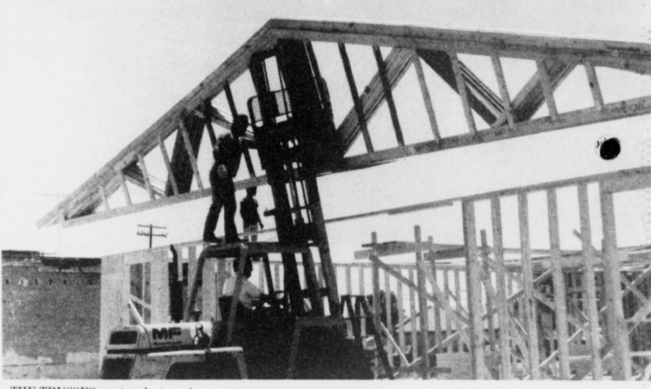
THE TRUSSES went up last week on the new post office in Bogata. Completion of the building is expected to be July 1. (Staff Photo by Mollie Williams)
