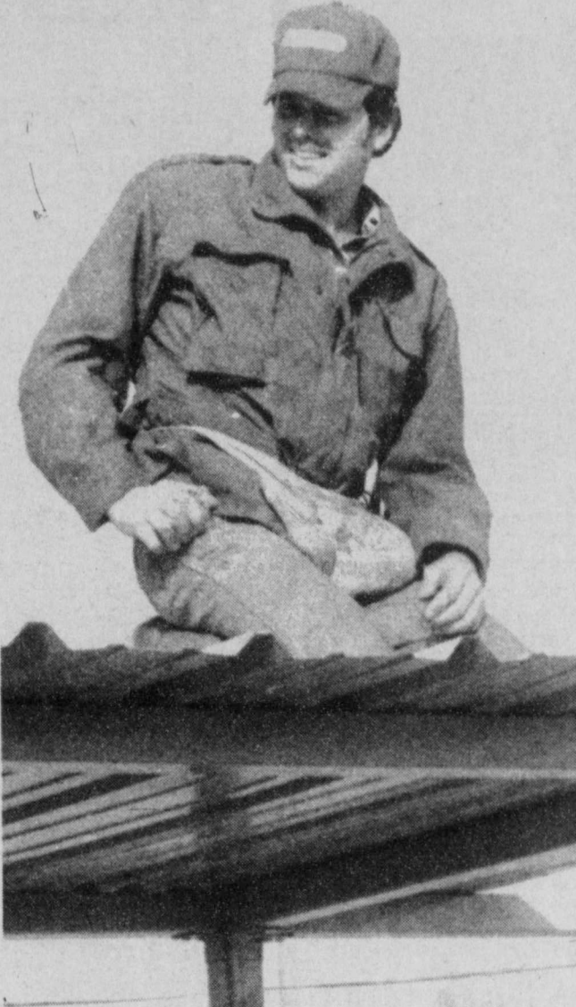
COVERED WALKWAYS on the Bogata campus are almost completed. The walkways connect the Junior High building to the Elementary building and cafeteria. Shown working on the roof is Darold Kuhlengel and on the ground is Marty Daniell. (Staff Photo)
