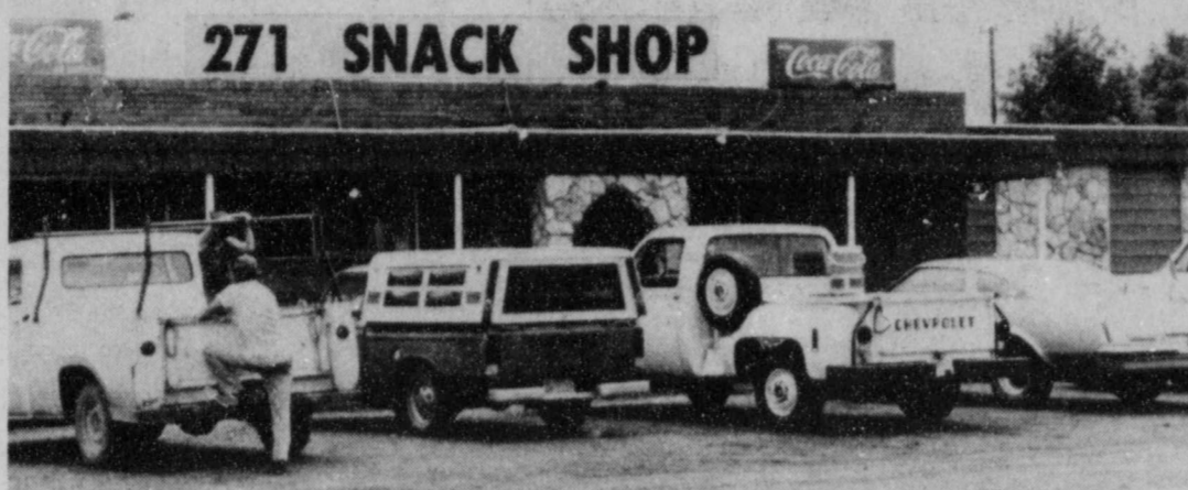
REMODELED—271 Snack Shop in Talco has undergone a face lift recently with a new front and covered walk. Native rock was used for accent and for the doorway. (Staff Photo).
