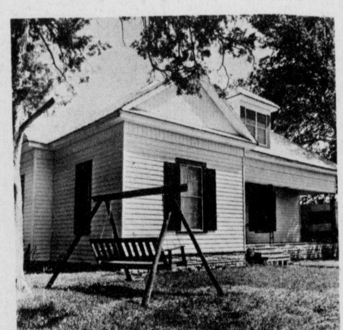
AFTER— After the installation of the U. S. Steel aluminum siding on the home the difference in the appearance is obvious.
