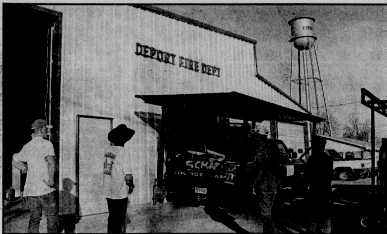
BACK UP -Members of Donald Day and Sons Metal Construction look at the newly replaced letters for the Depot Fire Station after they placed them on the newly remodeled and expanded station. The expansion is being paid for by fundraising by the Volunteer Fire Department, and provides a bay for the water tanker, which has been sitting out in the weather for some time now, much needed storage space and larger bay opening for the larger truck which barely fit in the older side of the station. (Staff Photo by Nanalee Nichols)
