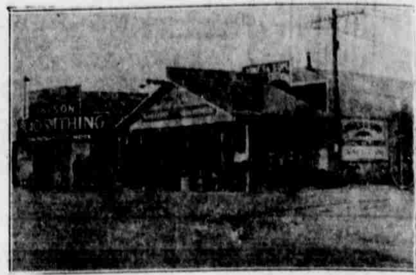
PICTURED ABOVE is the early day business operations of Jones and Son just off the southwest corner of the square. Jones & Son Sheet metal, recently sold to Al Fancher, operated in this location for over 50 years.
