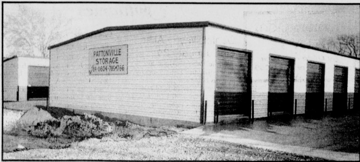
NEW STORAGE UNITS are open in Pattonville. The units are owned by Lorin and Kerry Murdock of Pattonville and are located on Highway 271 South. Thirty-two units are 10'x15' and were built by Donald Day & Sons Construction. They are the first mini-units available in Pattonville.
