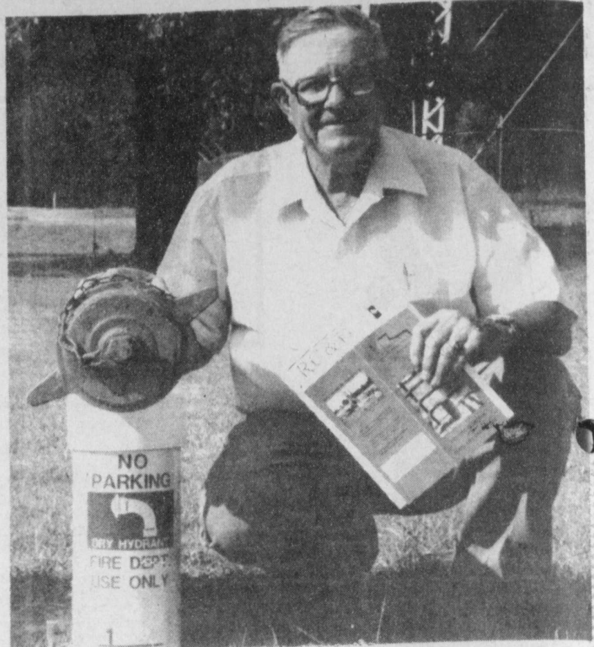
FEATURED FIRE PLUG! Deport Mayor Charles Foster is shown here with Deport's dry fire hydrant, which was installed last summer and was one of the first of its kind. The hydrant has been featured in a color brochure published by Resource Conservation and Development (RC&D). The brochure explains the uses and installation of a dry
