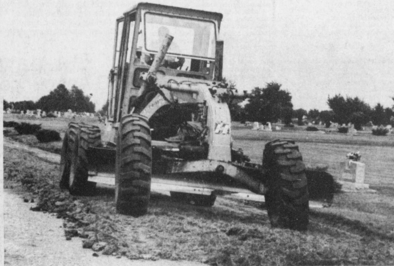
WORK-Highland cemetery roads are being grade and created in preparation for a gravel surface. (Staff Photo by Thomas Nichols)
