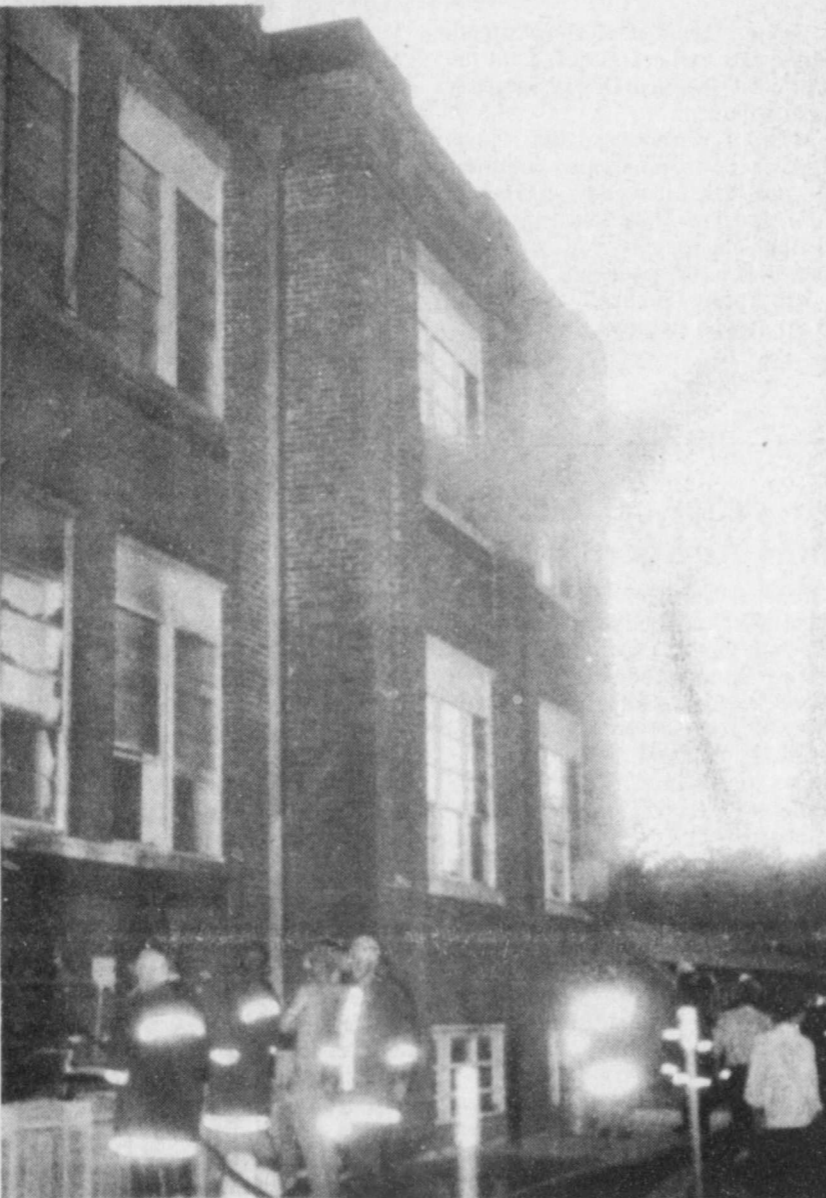
HEAVY DAMAGE -The Blossom Elementary School received heavy smoke and water damage, and the basement fire damage, after vandals ransacked the building, then lit fires in the basement and classrooms Sunday afternoon. School officials hope to have things back to normal by early December, and classes continue meanwhile in the gym. (Staff Photo)
